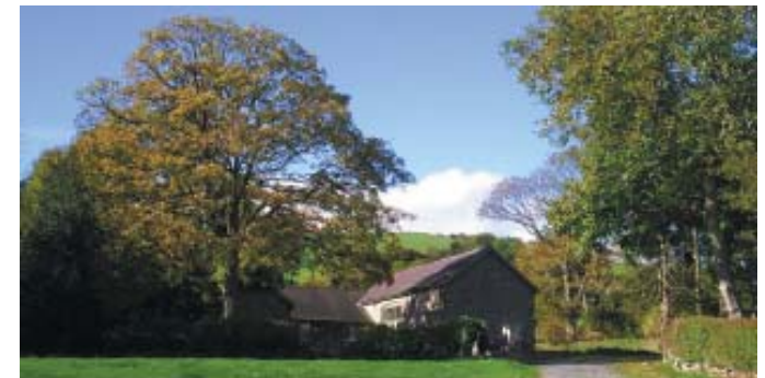
ABOVE The Hall Barn at the Bleddfa Centre. FAR LEFT A Map of the Place of the Wolf (detail), by Andrea McLean
